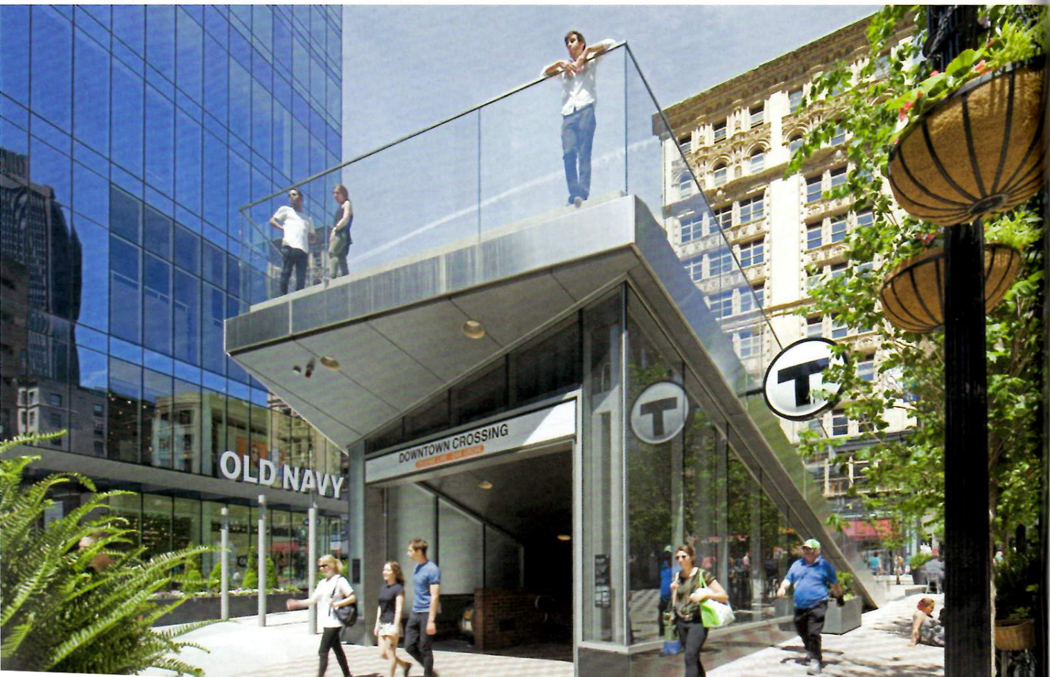
A new subway entrance design that doubles as an amphitheatre at the plaza level (Photo: John Horner ©.)
