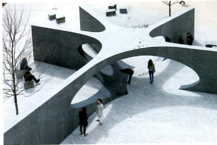
Figure 1.1 The memorial assembles 33 blocks of solid granite into a unified structure forming a shallow vault buttressed by five radial walls.
