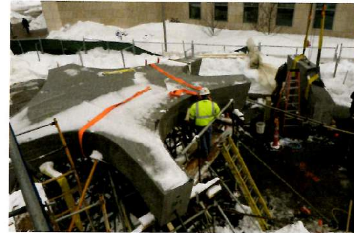
Figure 1.9 As the stone blocks arrived on site, they were assembled sequentially from center to periphery, requiring the five-sided keystone to be “placed” first as the supporting buttresses were built around it.
